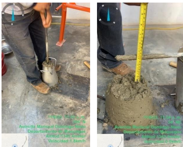
Figura 40. Slump de concreto fast-track.
