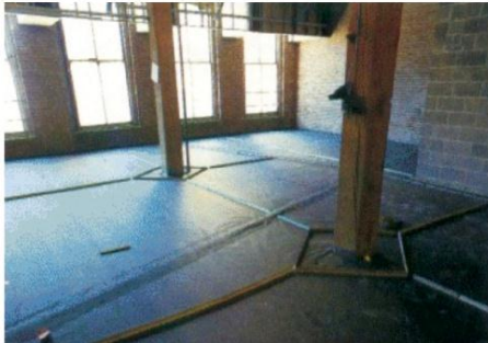
Fig. 5.2.3—Crack control strips.
