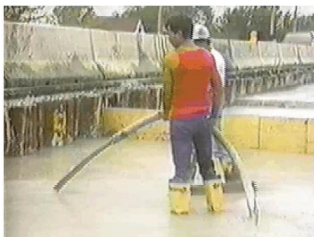
Fig. 5.1.2—Flowability of cellular concrete (video courtesy of Elastizell). See related video at http://www.concrete.org/Portals/0/Files/Media/ACI_523.3_Figure_5.1.2_Self-Leveling.mp4
