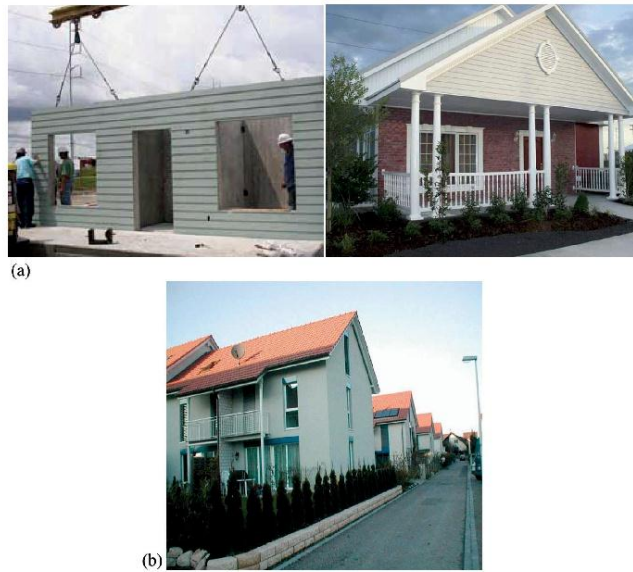
Fig. 10.4—Application of cellular concrete in residential construction: (courtesy of: (a) TAG Crete [2014]; and (b) Neopor [2012])
