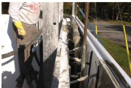
Fig. 5.1.1—Reusable formwork for a wall panel
