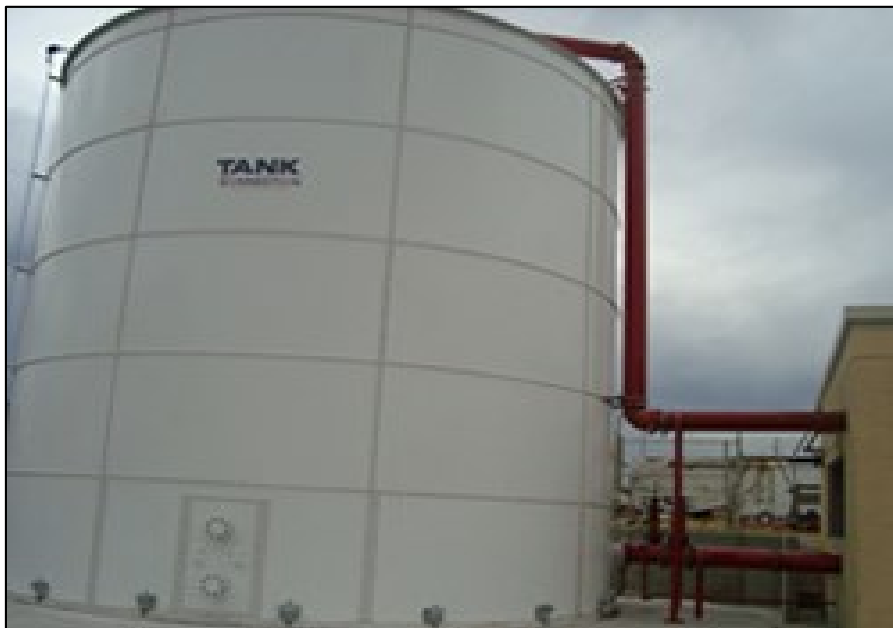
Figura 2, Tanque vertical. (tank connection, 2015)
