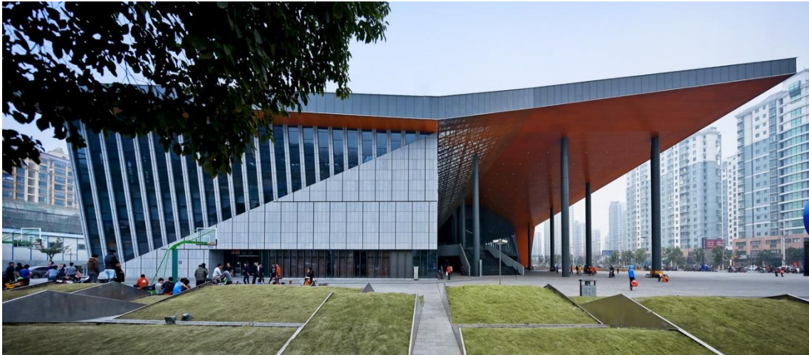
Figura 25. Centro de Deportes y Cultura Zhoushi. Recuperado de: https://www.archdaily.co/co/02-359464/centro-de-deportes-y-cultura-zhoushi-udg-yangzheng-studio/5361a56ac07a80f0d9000038-zhoushi-culture-and-sports-center-udg-yangzheng-studio-photo?next_project=no
