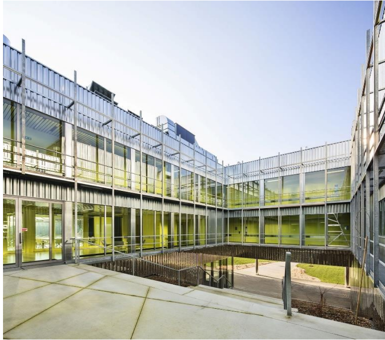
Figura 26. Vista exterior del atrio principal del BIOPOLE, Bussinees icubator Nota. Fuente: Archdaily, 2015. Obtenido de: https://www.archdaily.com/614117/biopole-biotech-business-incubator-peripheriques-architectes
