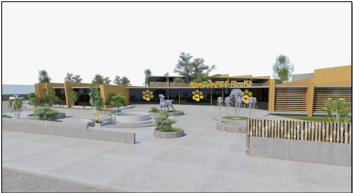
Vista exterior – Fachada principal
