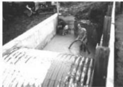
Fig. 7.4—Geotechnical fill around steel culvert under existing bridge.
