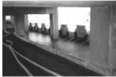
Fig. 7.1—Geotechnical application under a bridge structure with mechanically stabilized earth (MSE) containment walls.
