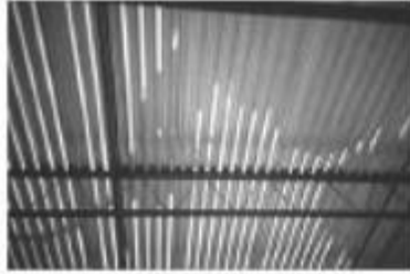
Fig. 6.1—Casting cellular concrete over vented steel deck.
