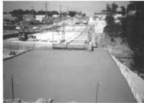
Fig. 7.3—Geotechnical roadway base at bridge approach.
