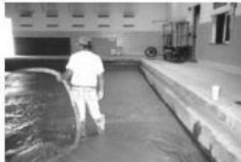
Fig. 7.5—Filling abandoned swimming pool with low-density concrete.
