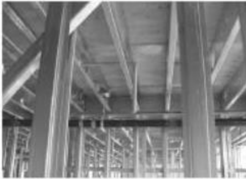
Fig. 6.4—Wood frame roof deck substrate from below.
