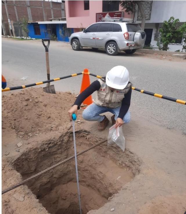
IMAGEN 05: CORROBORAMOS QUE LA MEDIDA SEA LA CORRECTA Y LLEGAMOS A 1,70M
