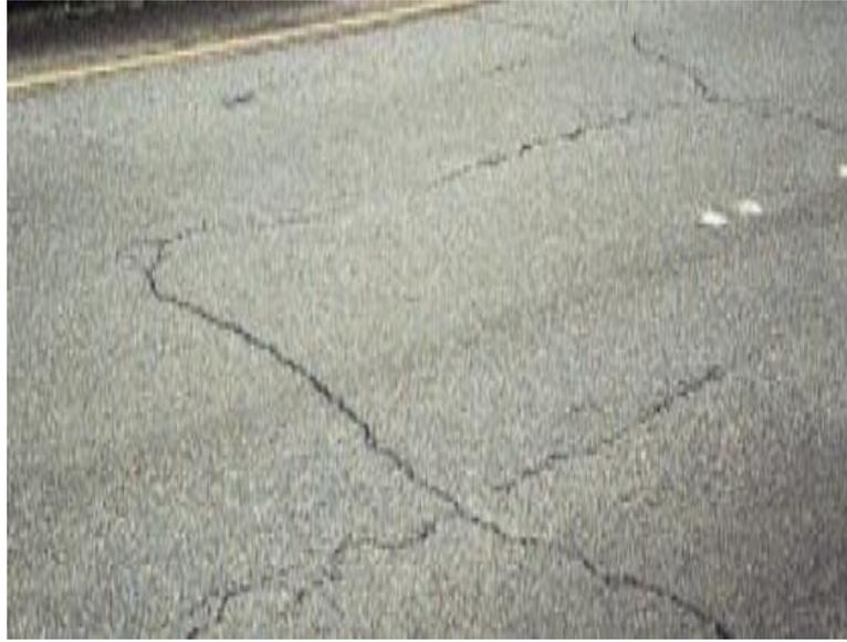
*Figura 5: Agrietamiento en bloque. Fuente: Pavement Surface Condition Field Rating Manual for Asphalt Pavement. Washington State, 2013.*
