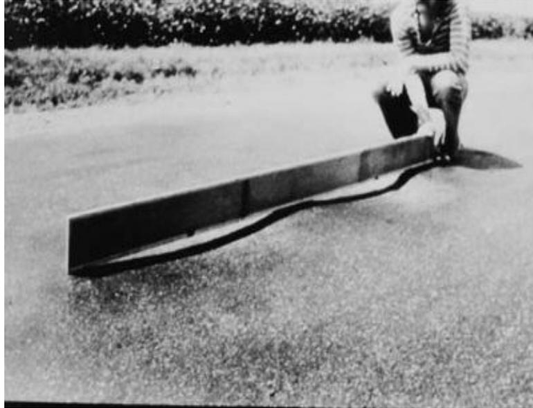
*Figura 7: Corrugación. Fuente: Standard Practice for Roads and Parking Lost Pavement Condition Index Surveys. Pennsylvania, 2016.*
