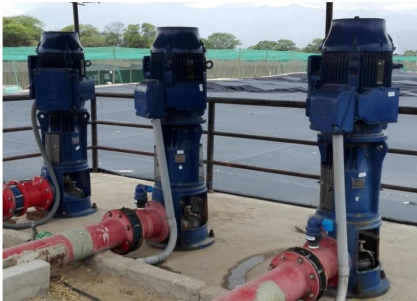
*Figura 8:* Bomba Turbina Vertical 50 HP
