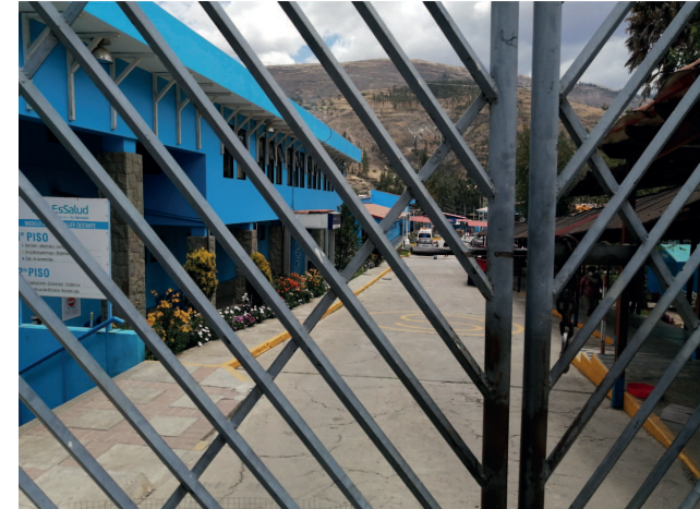
Interior del Hospital II - Essalud
