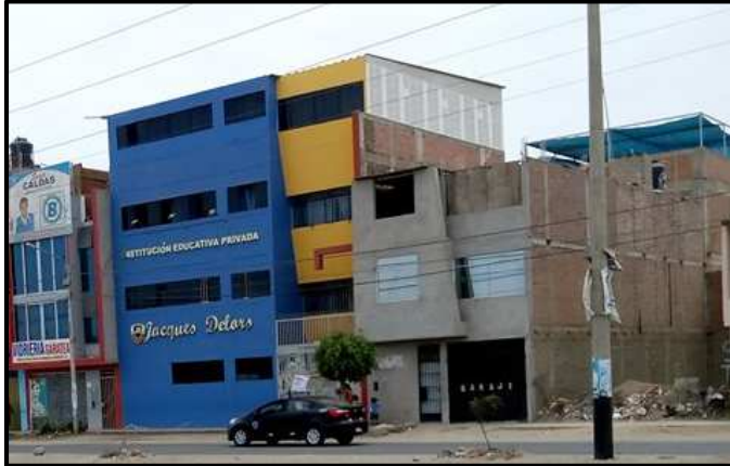
FUENTE: ARCHDAILY JAQUES DELORS – FACHADA PRINCIPAL
