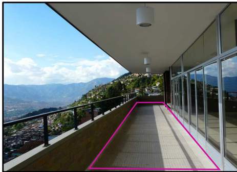
BALCON DE AULA MULTIPLE
