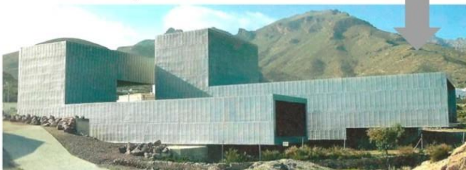
4. Paneles de aluminio perforado – 2.50m. X 0.80m.
