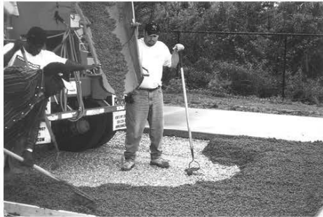
Fig. 8.1—Placement of pervious concrete by rear-discharge mixer truck.
