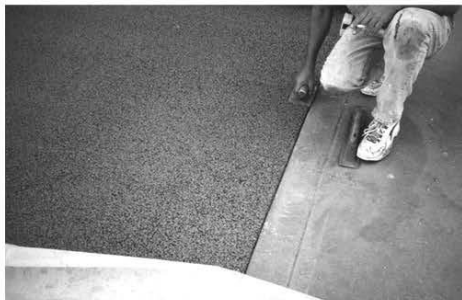
Fig. 8.10—Edging pervious concrete to improve appearance of corners.
