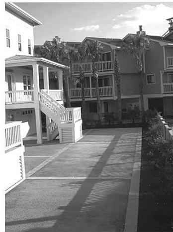
Fig. 3.1—Parking lot built with pervious concrete pavement.
