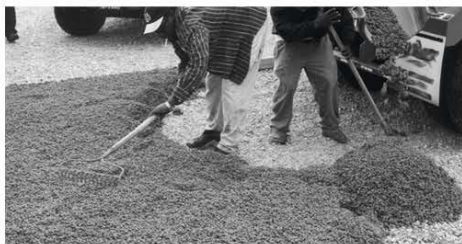
Fig. 8.3—Raking pervious concrete to rough elevation.
