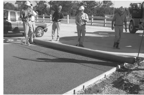
Fig. 8.7—Example of compaction of pervious concrete by rolling.
