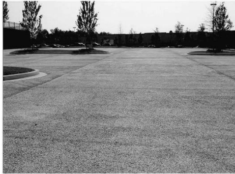
Fig. 12.3—Pervious concrete parking lot.
