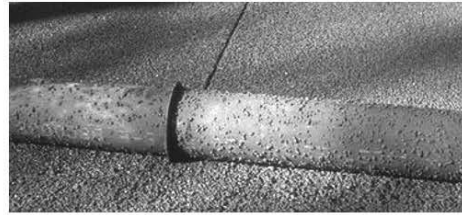
Fig. 8.12—Example of jointing tool built into primary roller.
