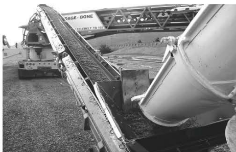
Fig. 8.2—Use of conveyor to place pervious concrete.
