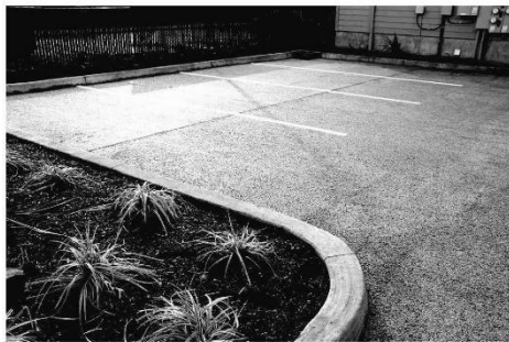
Fig. 12.4—Pervious concrete parking area.
