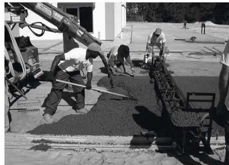
Fig. 8.5—Use of vibratory screed for strike off of pervious concrete.
