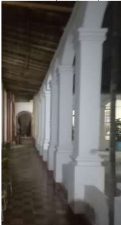
Columnas patio principal
