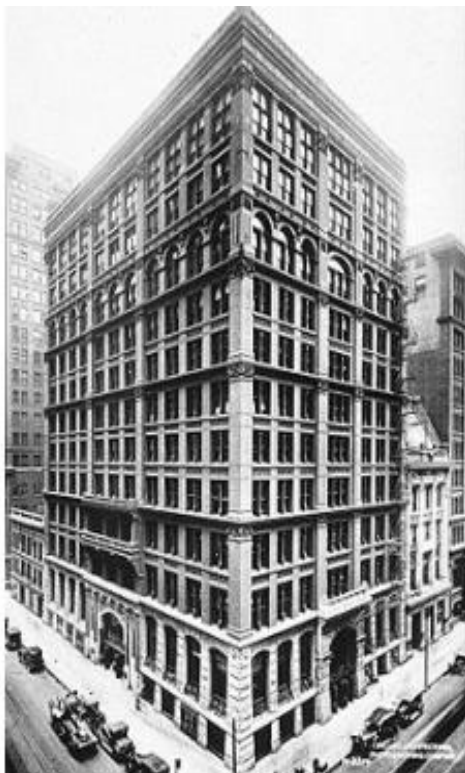
Figura 4: Edificio Home Insurance.
