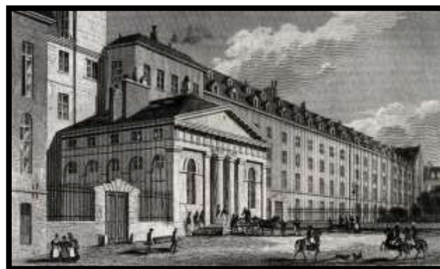
Figura 64: Hospital Hotel Dieu
