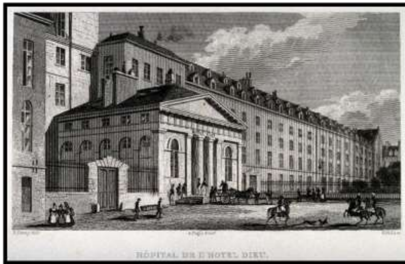
Figura 52: Hospital Hotel Dieu
