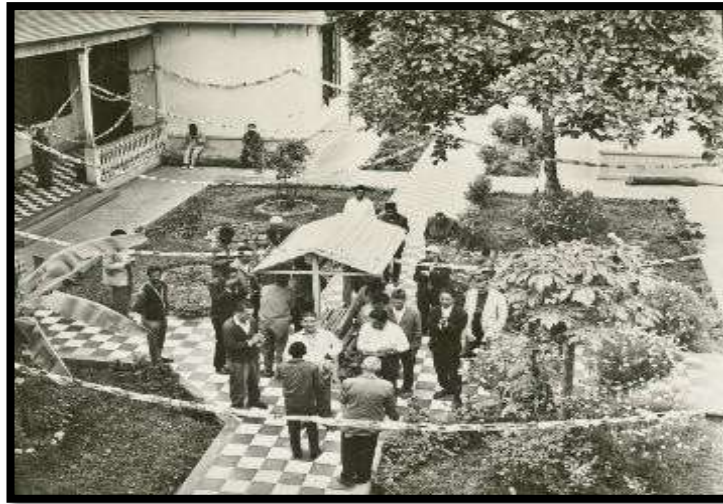
Figura 39: Patio Central – Hospital Larco Herrera
