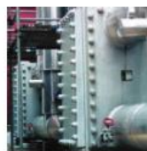
Vertical Compabloc for liquid/liquid heat recovery
