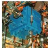
Suspended mounting for condensation duties
