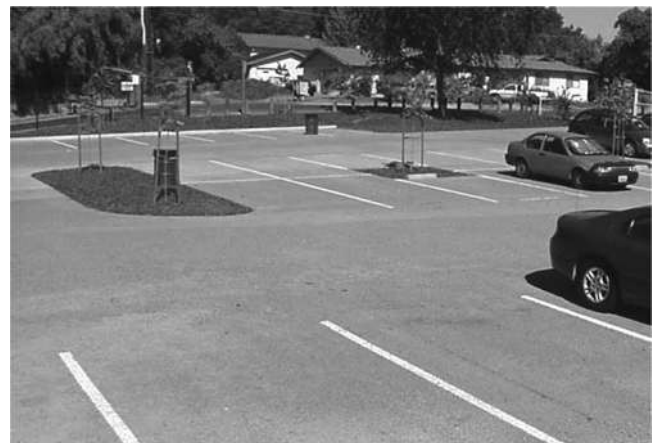
Fig. 12.1—Pervious concrete stormwater management system.
