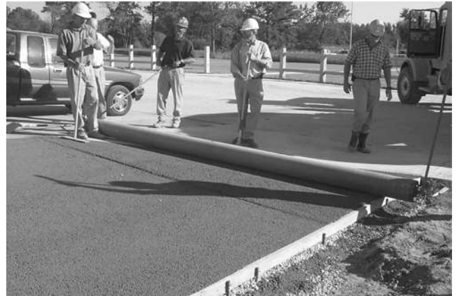
Fig. 8.7—Example of compaction of pervious concrete by rolling.
