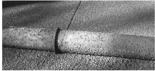
Fig. 8.12—Example of jointing tool built into primary roller.
