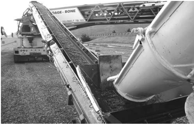
Fig. 8.2—Use of conveyor to place pervious concrete.
