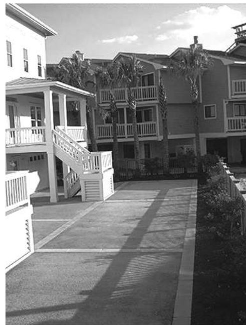
Fig. 3.1—Parking lot built with pervious concrete pavement.
