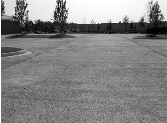
Fig. 12.3—Pervious concrete parking lot.
