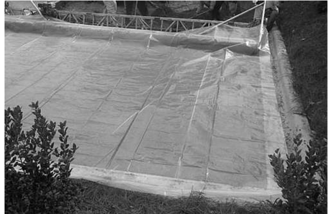
Fig. 8.13—Demonstration of curing with plastic sheeting immediately after compaction
