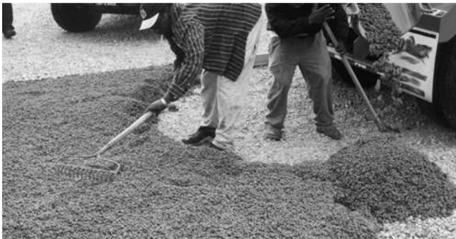
Fig. 8.3—Raking pervious concrete to rough elevation.
