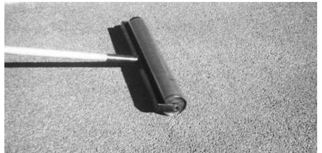
Fig. 8.8—Example of small roller used for compacting small paved area.
