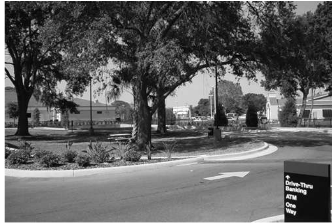
Fig. 3.2—Pervious concrete pavement used within the drip line of tree.
