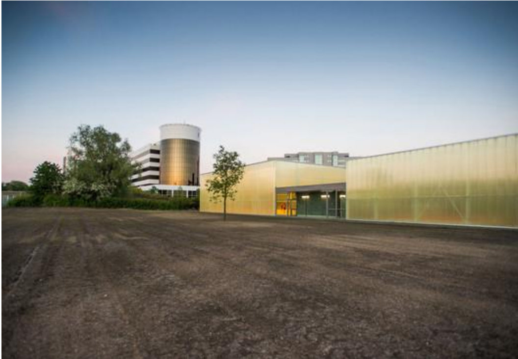
Figura 22. Centro Deportivo Kiel. Recuperado de: https://www.archdaily.pe/pe/758296/centro-deportivo-architects/54640c5ce58ecee5000115-ur_sck_foto_03-jpg
