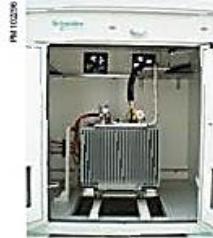
Transformer in PV box
