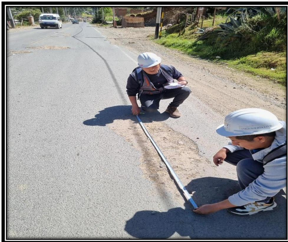
➤ IMAGEN 2: MEDICION DEL ANCHO DE CALZADA DEL PAVIMENTO FLEXIBLE
