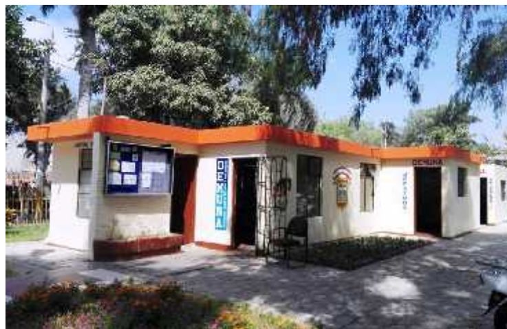
Figura 3. Vista principal de la DEMUNA - Chiclayo
