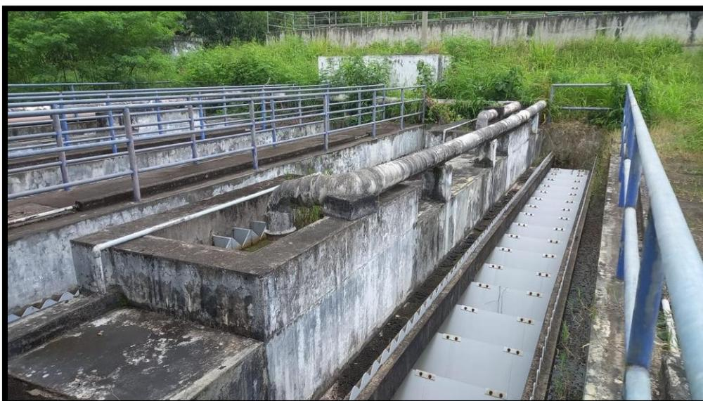
**Figura 23: Reactor anaeróbico -PTAR Santa Ana**
