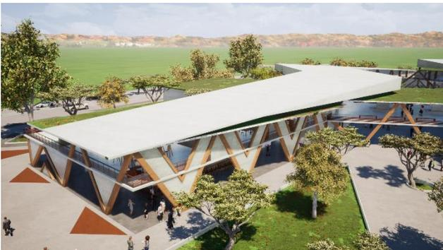
**TECHOS DE ESTRUCTURAS METÁLICAS CON COBERTURA ONDULINE.**
