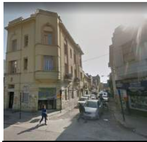
Calle interior 2 Trieste (vehicular – peatonal)
