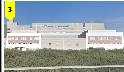
KEISER PERMANET ORANJE COUNTY (HOSPITAL)
