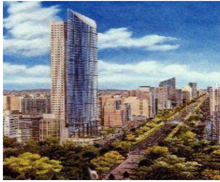
Figura 3. Torre Mayor – México
