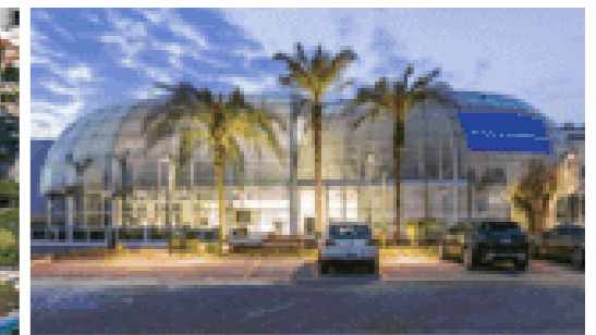
Reforma del Hospital Moriah
