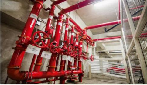
A photograph showing a complex network of red pipes and valves, likely part of a fire water and foam suppression system, installed in a utility room or basement.                                           |
