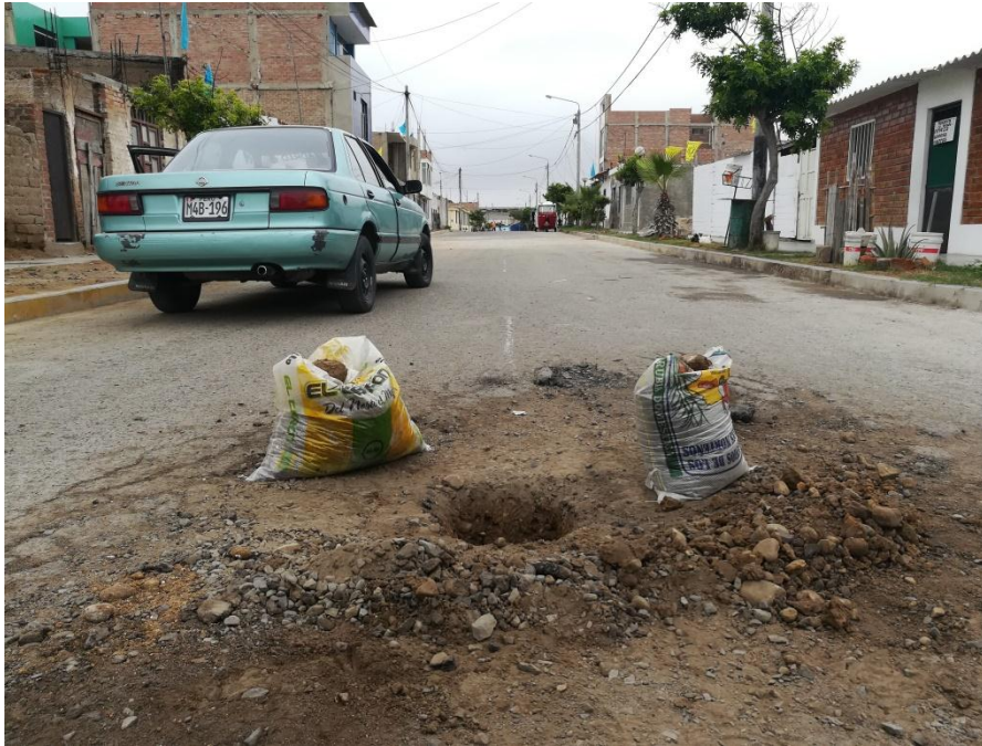
Calicata 2 - Ca. Juan Fanning.
