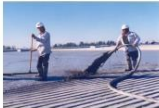
Fig. 1.2—Roof deck application (click on picture to view video).
