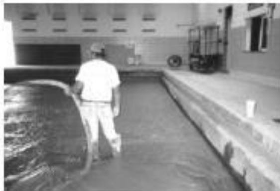
Fig. 7.5—Filling abandoned swimming pool with low-density concrete.
