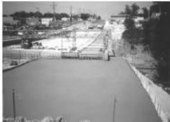
Fig. 7.3—Geotechnical roadway base at bridge approach.
