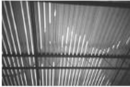
Fig. 6.1—Casting cellular concrete over vented steel deck.
