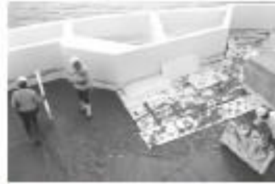
Fig. 6.2—EPS insulation board placed in cellular concrete slurry over structural concrete deck.
