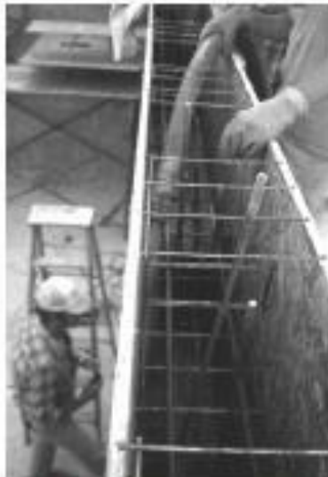
Fig. 7.7—Cellular concrete as wall fill with stay-in-place forms.
