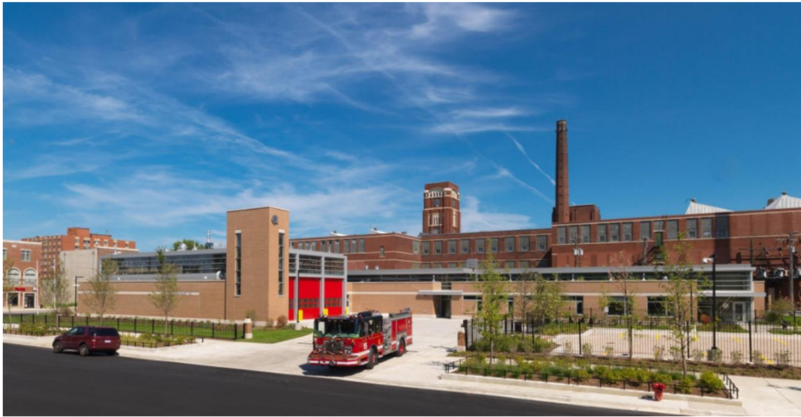
Figura 15: Estación de bomberos tipo III. Recuperado de: https://www.archdaily.pe/pe/625648/compania-de-bomberos-no16-dlr-group/53e2f88dc07a80bf02000344-engine-company-16-firehouse-dlr-group-image?next_project=no
