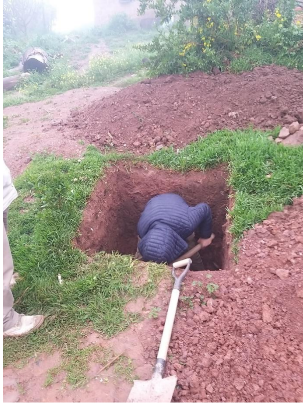
Figura 9: Calicata in situ C-01
