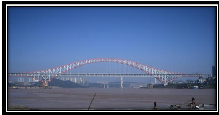
Figura 1: Puente Chaotianmen, China, 2009
