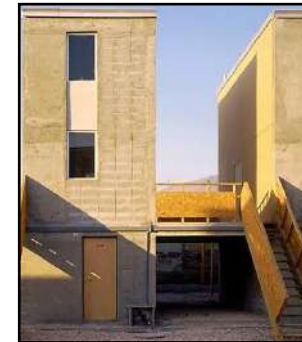
FACHADA Fuente: https://archdaily.pe
