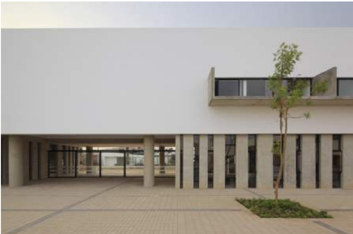
Figura 5. Vista interior 2 Colegio LVC.
