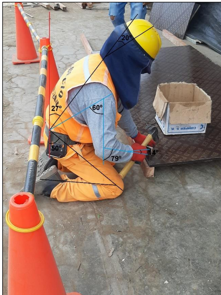
Figura 20: Armado de paneles (RULA – T1), Consorcio Negrón, 2021.
