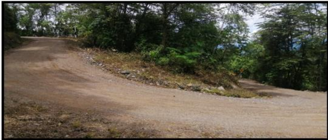
PI 154 (progresiva 05+378.28), radio = 9.26 m.
