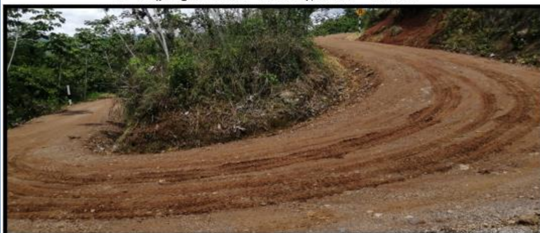
PI 55 (progresiva 02+229.62), radio = 8.12 m.
