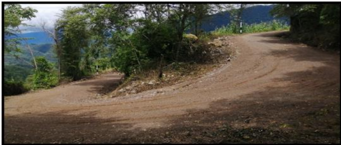
PI 169 (progresiva 05+821.70), radio = 7.16 m.
