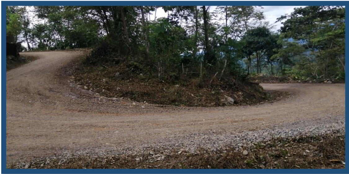
PI 198 (progresiva 06+780.88), radio = 8.07 m.
