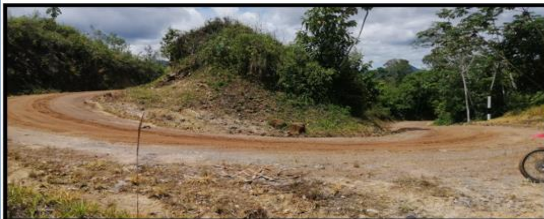
PI 41 (progresiva 01+862.85), radio = 8.17 m.
