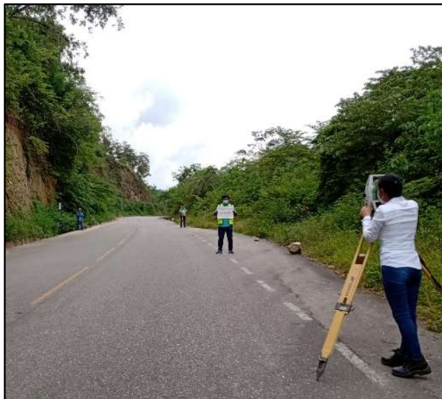
Figura 17. Km. 4+000.00 al Km. 5+000.00
