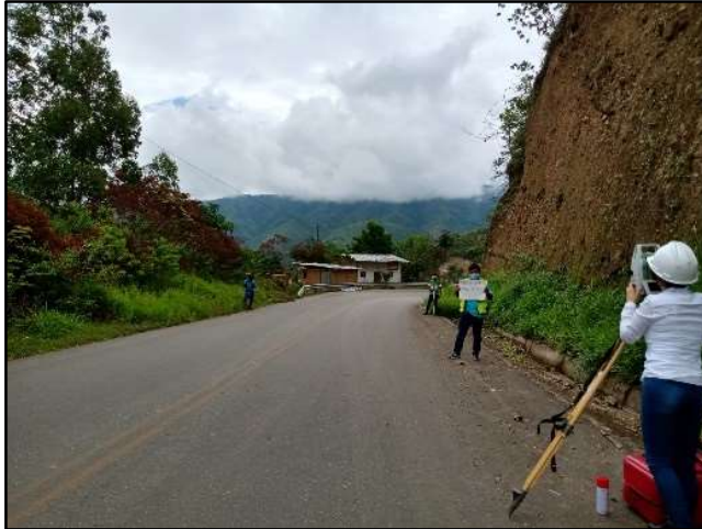
Figura 16. Km. 3+000.00 al Km. 4+000.00
