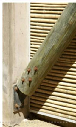
**ANCLAJE DE LA ESTRUCTURA**
