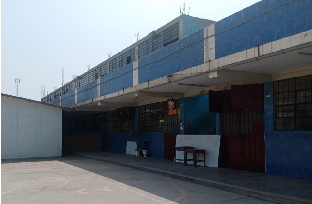
Figura 13: Irregularidad por out of plane setback.
